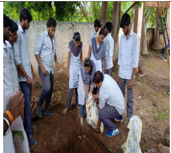
NSS Volunteer Students Digging Soak Pit
