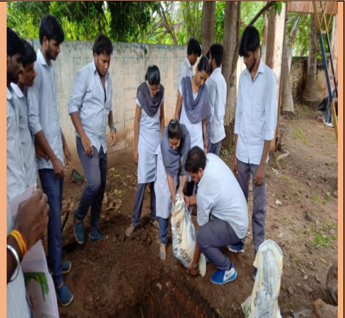
NSS Volunteer Students Digging Soak Pit
