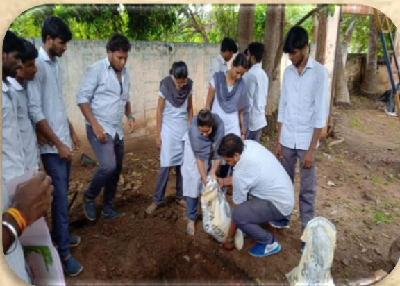
NSS Volunteer Students Digging Soak Pit
